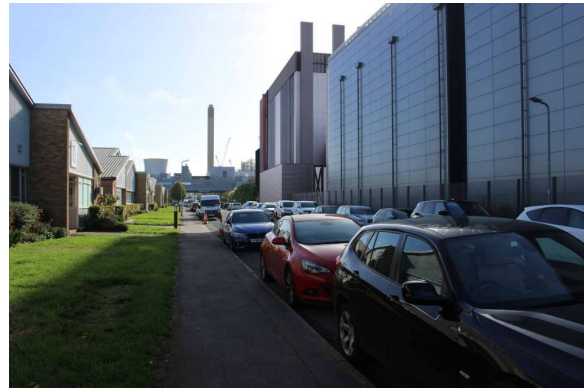
Above: proposed image of the application site from the west in Banbury Avenue (1).
